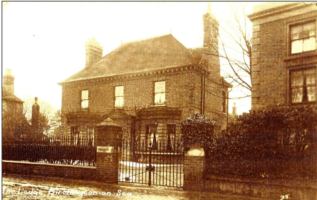
The Lodge – Canterbury Road c. 1920
